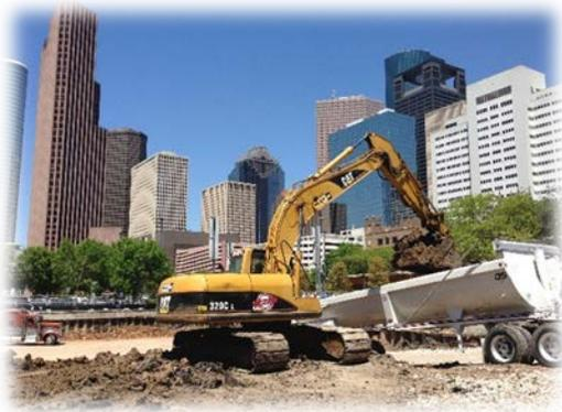
The use of innovative source-area excavations has gained popularity due to the assurance that all environmental contaminants can be permanently removed and rapid closure is possible. MEC<sup>x</sup> has designed and developed techniques for excavating contaminated soils from beneath occupied buildings and active facilities.
